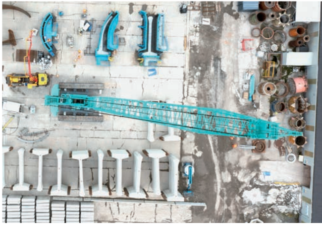
G H Johnson's CKE800G-3 and CKE2500G-2, working at Stanton Precast's factory in Ilkeston, Derbyshire, are helping deliver over 13,000 pre-cast concrete segments for three of HS2's tunnels.
